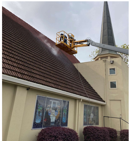
Church roof steam cleaned
