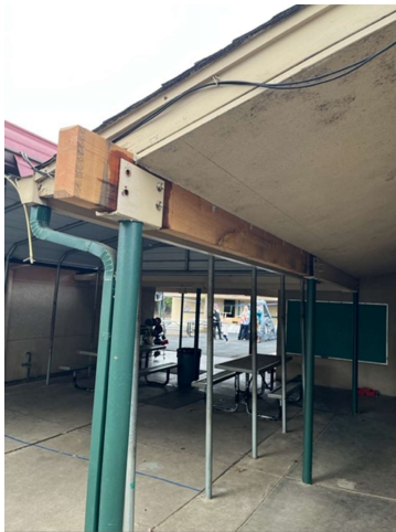
Repaired dry rotted beams
